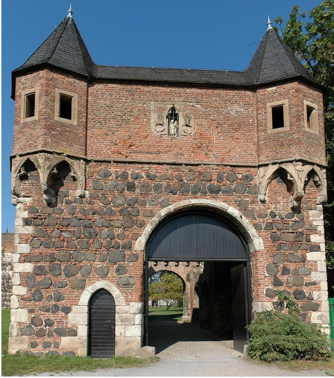
Figure 1: An example of a wicket gate [32], to the left of the main gate, used in the Middle Ages to provide fine-grain access to city or castle gates.
